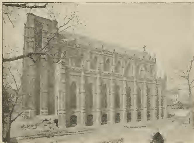
ST. FINBAR CATHEDRAL, BEING REBUILT.
